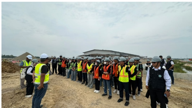
Safety briefing for the visitors from POLNEP before their tour of the Rembus Depot site
